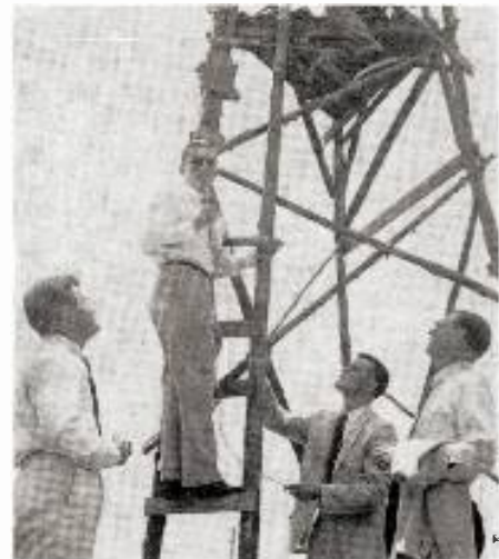
WITH the dedication of its new radio color tower, WBT Charlotte has advanced another step in its assault on new electronic frontiers. Forsaking steel and chromium trappings for Tarheel ingenuity, WBT was able to adapt an old windmill as its radio color transmitter. The equipment and site were donated by a listener after he heard disc jockey Owen Spann (mounting tower) announce plans for broadcasting fights in black and blue, royal broadcasts in purple and hillbilly music in tobacco brown. Charlotte Mayor Jim Smith (right) officially dedicates the new gear as local newspaper reporters cover the event.
